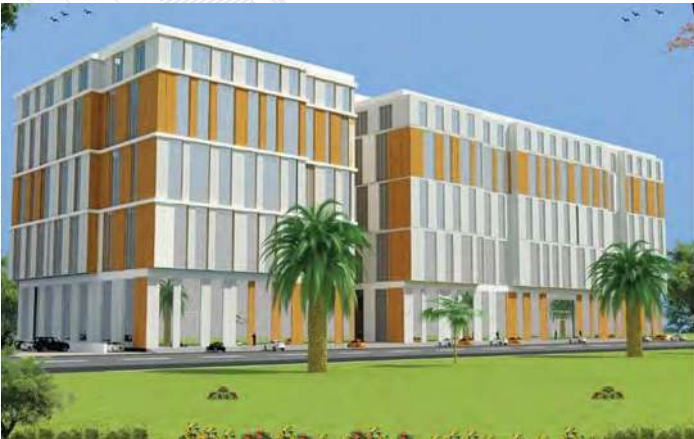
Project : Residential Commercial Building @ Azaiba. Consultant : Abdullah Mukadam & partners LLC. Area : 62000 M 2
