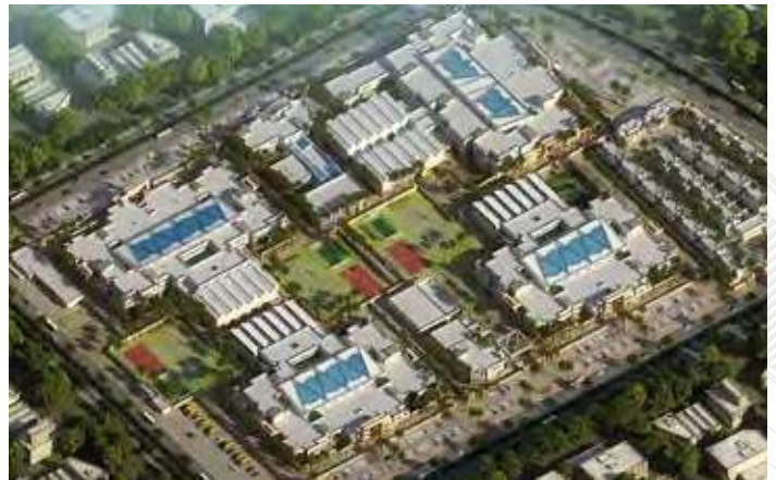
Project : Al Andalus School Complex @ Al Kheesa Umm Salal, Qatar. Consultant : Dimesnions Engineering Consultants - Qatar. Area : 54,036 M 2
