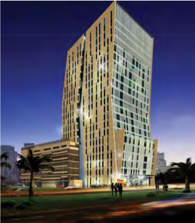
Project : Commercial Tower - Qatar. Consultant : Al Sraiya Engineering Consultant - Qatar. Area : 33,000 M 2
