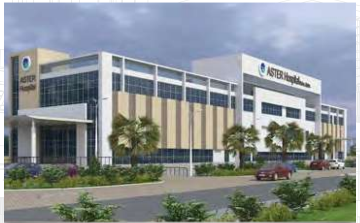
Project : Aster Hospital , Old Airport. Consultant : Dimesnions Engineering Consultants - Qatar. Area : 4,700 M 2
