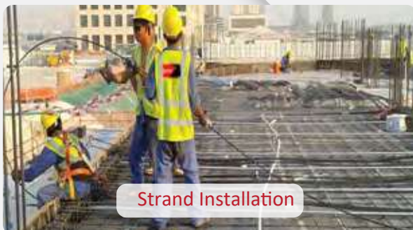
Completion of Bottom Steel
