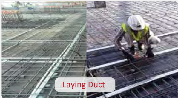
Tendons Marking at bottom shuttering
