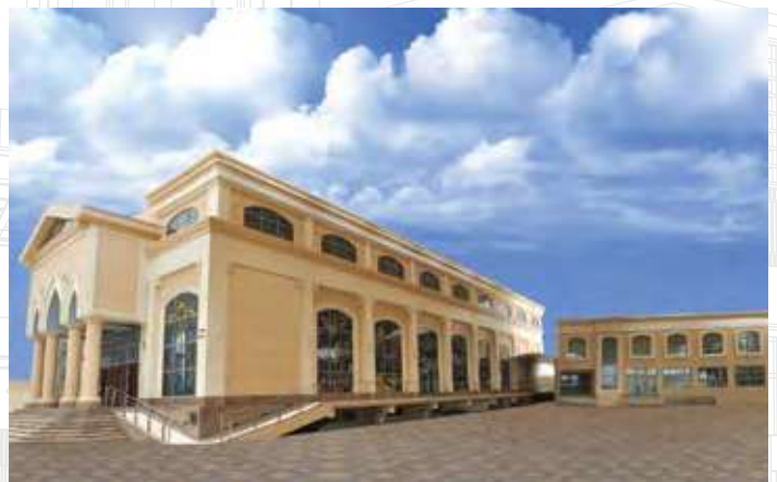
Project : Catholic Church @ Salah. Consultant : Al Manarah Engineering Consultancy. Area : 1,500 M 2
