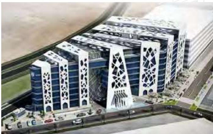
Project : Commercial Building @ Muscat Hill – OMINVEST. Consultant : Design Unit Engineering. Area : 44,000 M 2
