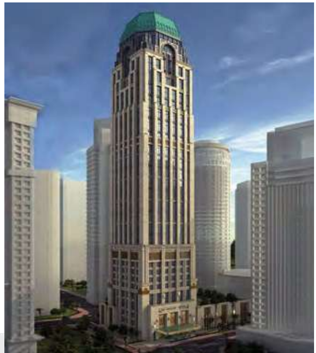
Project : Waldorf Astoria Hotel (3B+G+M+43). Consultant : Lacasa Architect & Engineering. Area : 65,000 M 2
