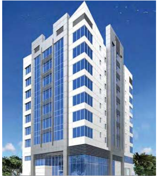
Project : Residential Building @ Najma, Qatar. Consultant : DCE Consulting & Engineering - Qatar. Area : 6,000 M 2
