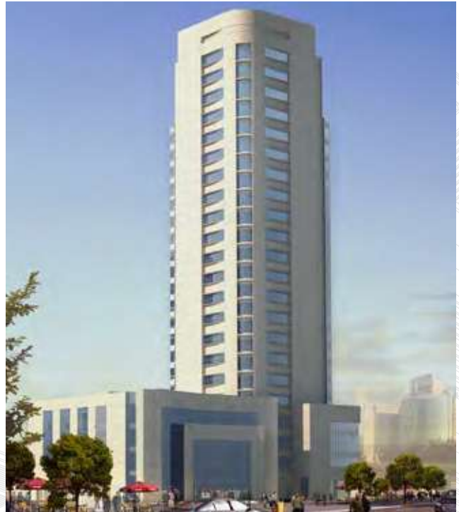
Project : Marina Tower, Com - 031. Consultant : EHAF Consulting Engineers. Area : 45,000 M 2
