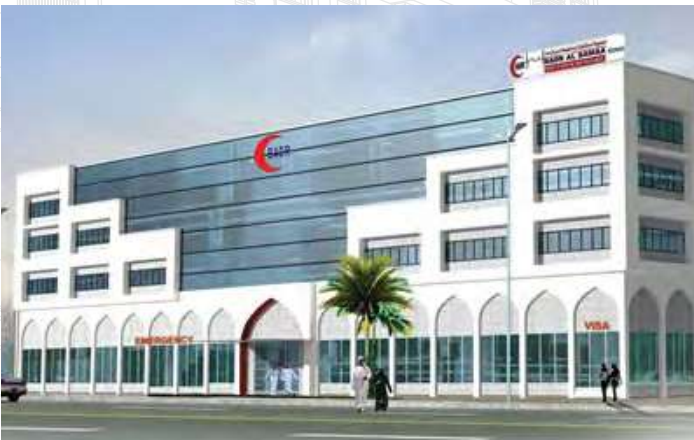
Project : Badar Al Sama Hospital @ Sohar. Consultant : National Engineering Office (NEO). Area : 7500 M 2
